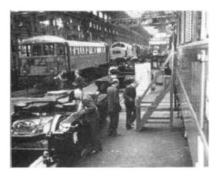
Members inspecting Locomotives under construction at the Vulcan Works of the English Electric Co. Ltd., Newtonle-Willows.
