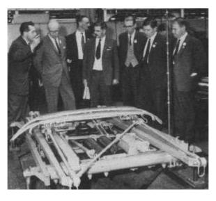
A group of members inspecting a crossed-arm pantograph, one of a batch supplied for British Railways 25kV a.c. locomotives, during the visit to AEI Ltd., Trafford Park, Manchester.
