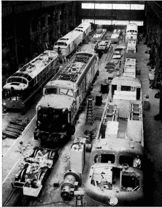
General View of Diesel Erecting Shop
