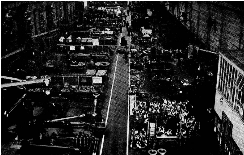
General View of Fitting Shop
