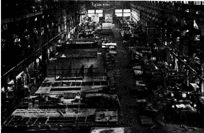
General View of Tender Shop showing Stages in Erection
