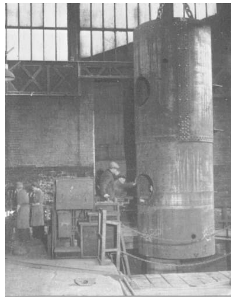
Rivetting Boiler Shell.
