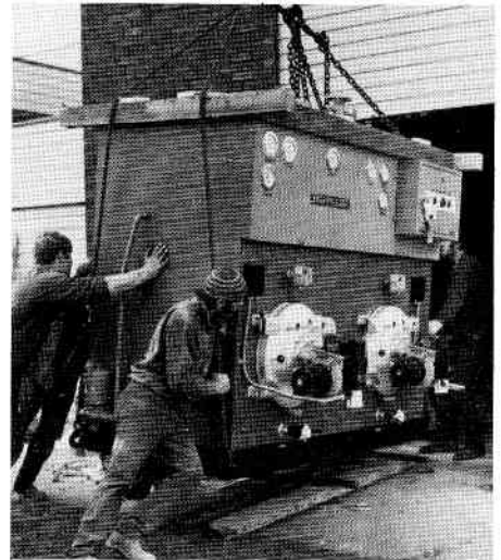
GEC Golcalor packaged boilerhouse being installed in R.C. School, Cheadle Hulme.
